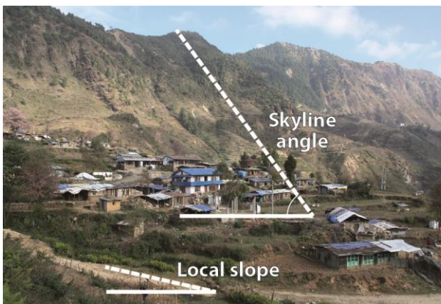
Figure 1. Landslide-prone houses in Sindhupalchok District, Nepal, showing the difference between the maximum angle to the skyline and the local slope of the ground surface.
